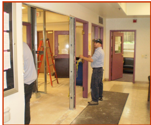
The Renovation in progress!
